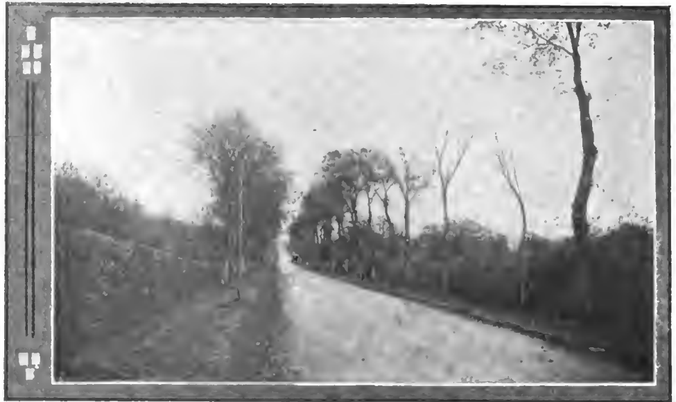
Illustrating Roads Building in France—Showing Tree Protection
